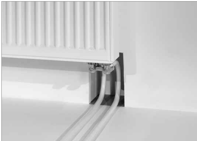
Radiator connection from the wall
