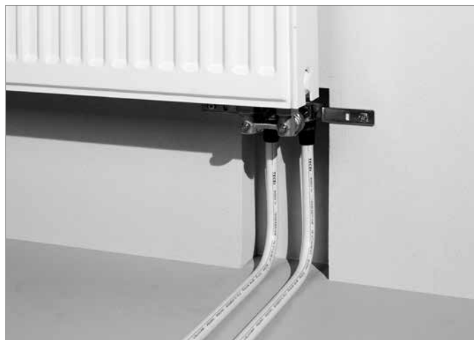
Radiator connection with radiator mounting unit, wall-mounting - connected to the valve block
