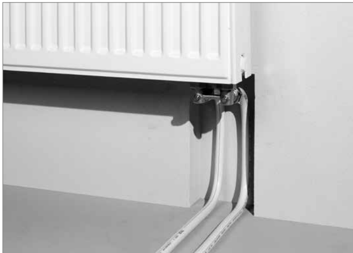
Radiator connection from the wall
