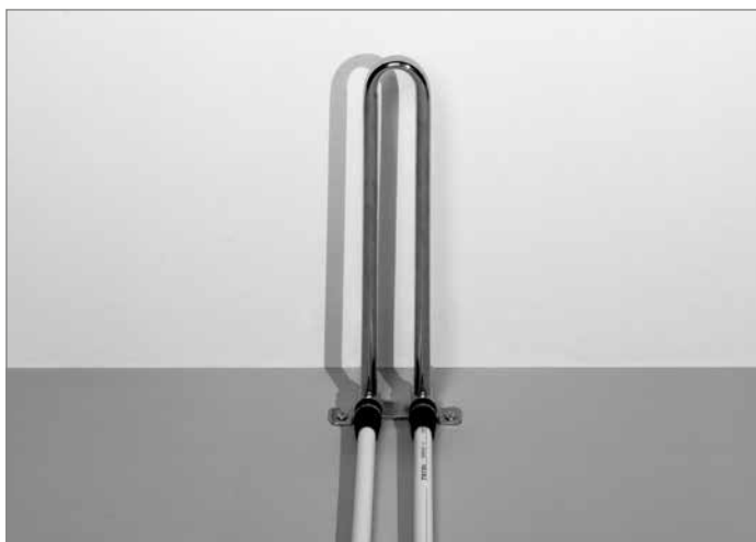
Radiator connection with radiator mounting unit, floor-mounting - ready to push free
