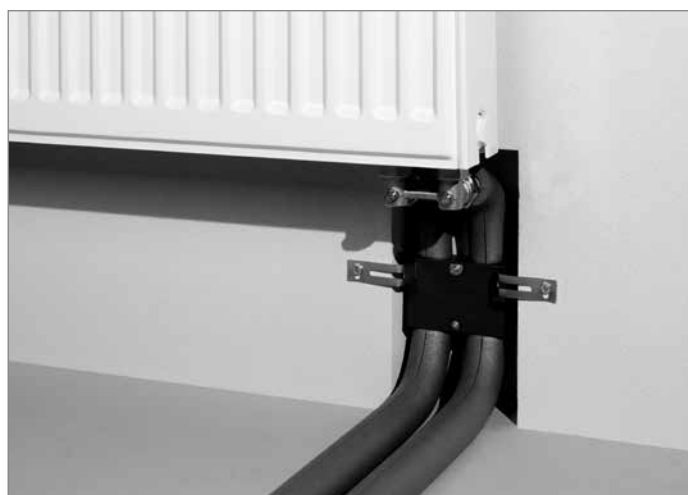
Radiator connection with mounting unit - connected to the valve block
