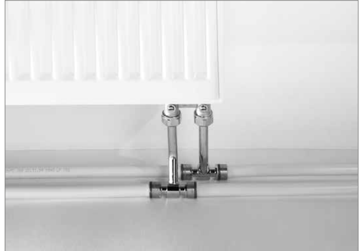
Radiator connection with radiator mounting tee
